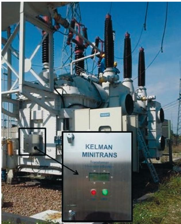
Fig. 2. Monitoring system of water and gas content in oil in 160 MVA autotransformer
